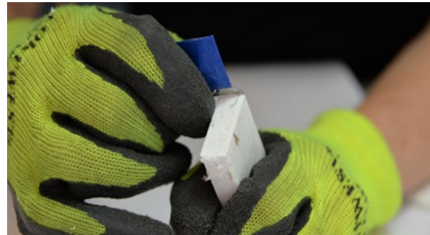
Use a Stanley knife blade to finish off the rough edge
