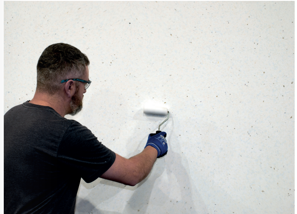
↑ Applying an FR treatment to a full sheet of Alba
