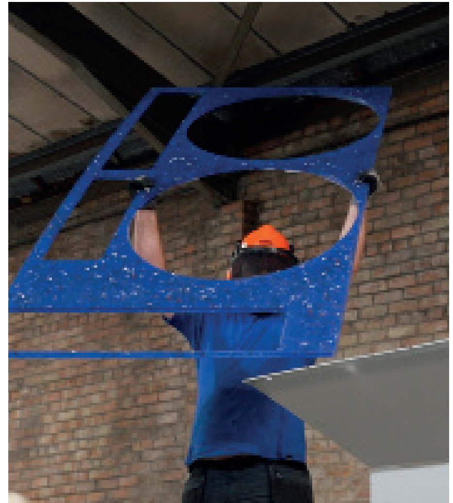
↑ In-house recycling of skeletal sheet waste
